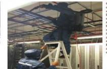
Cable trays, lighting, ductwork, and piping are all areas of your Data Center that are outof sight and often neglected. Not only do harmful dustparticles settle on the equipmen in the room, but also accumulate on the overhead components Building vibration and airflow changes can dislodge settled particular
